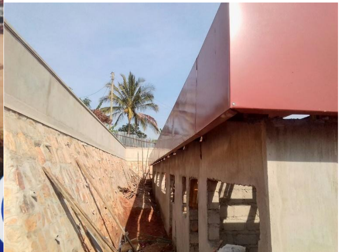
Station shop building works in progress
