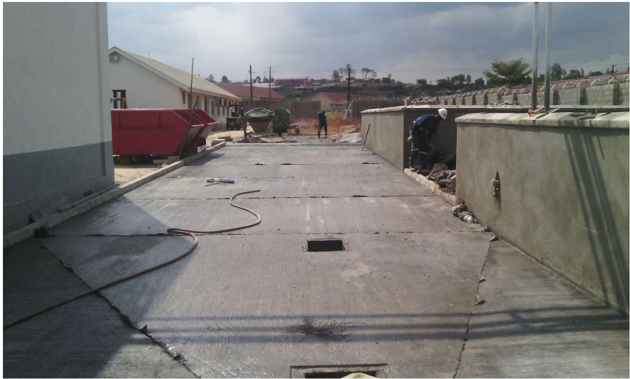
Class 35, 200mm thick drive way concrete slab, ready for use – Coca Cola Namave plant
