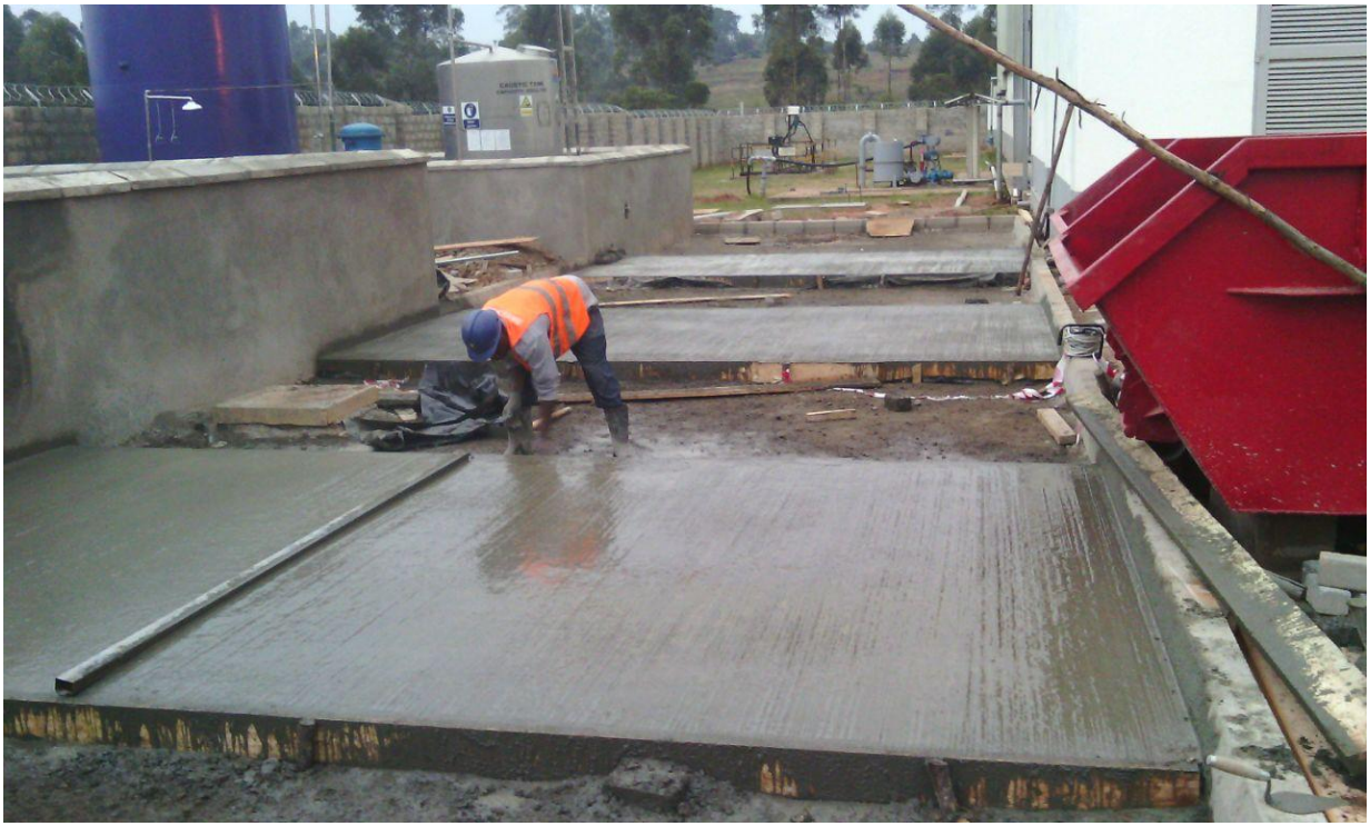
Class 35, 200mm thick drive way concrete slab – Coca Cola Namave plant
