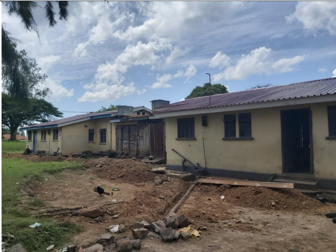
Refurbishment of NARO staff houses at NaSarri- Serere
