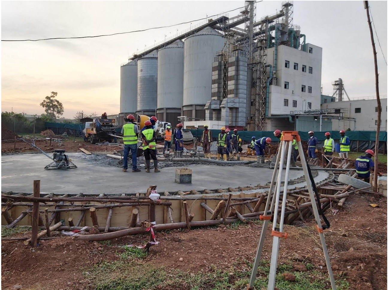
Class 35 Concrete works for calamity tank foundation at Nile Breweries Jinja Plant
