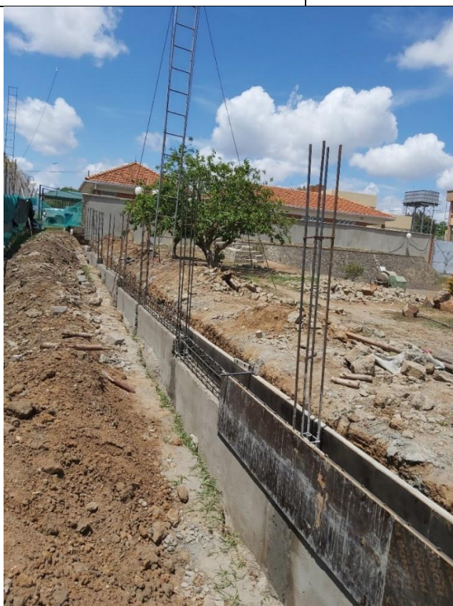
Perimeter wall ground beam works in progress - BOU Arua Branch.
