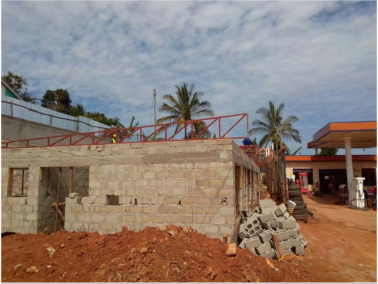
Fuel station shop and office building works in progress- Gaz Nabingo
