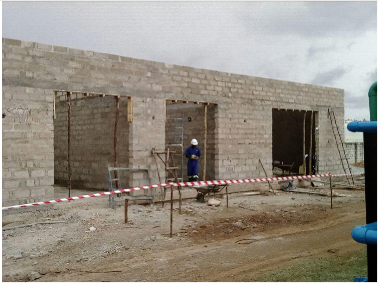
Equipment Room ready for roofing– Coca Cola Mbarara Plant
