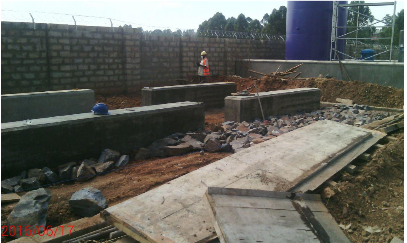
Concrete saddles (foundations) for horizontal above ground fuel tank – Coca cola Mbarara plant
