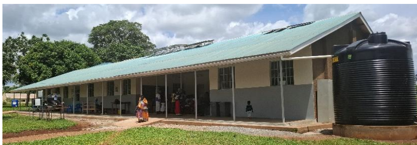
H C III Refurbishment
