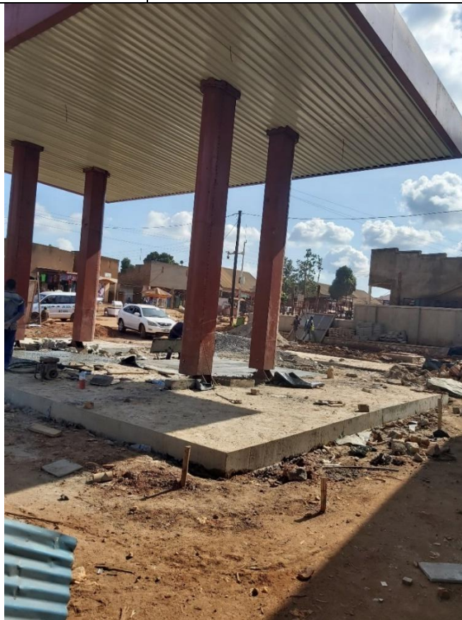
Construction of Oil Com Fuel station at Kireka- Mityana Road works in progress
