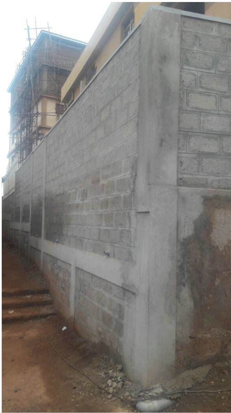
Three (03) meters high Retaining wall– Oilcom Sir Apolo Kagwa Road
