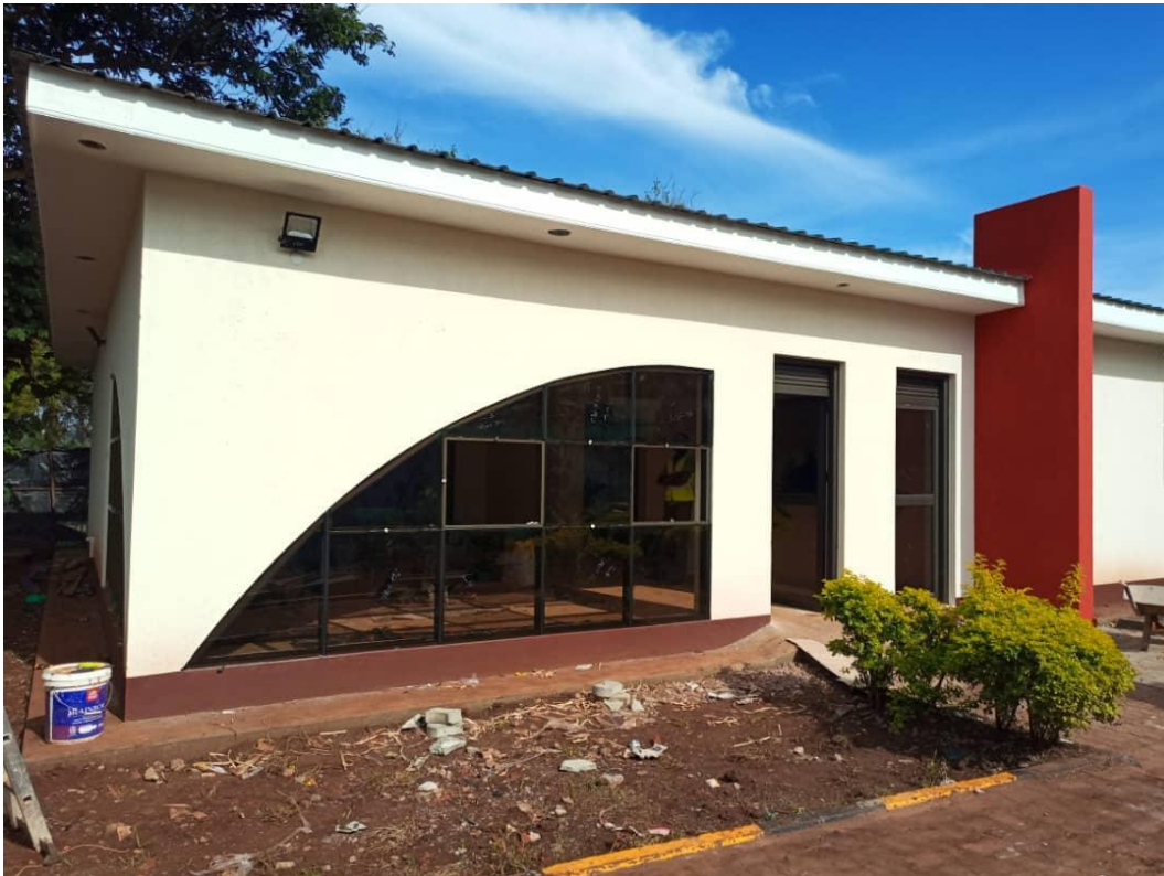
New Reception Building at NBL
