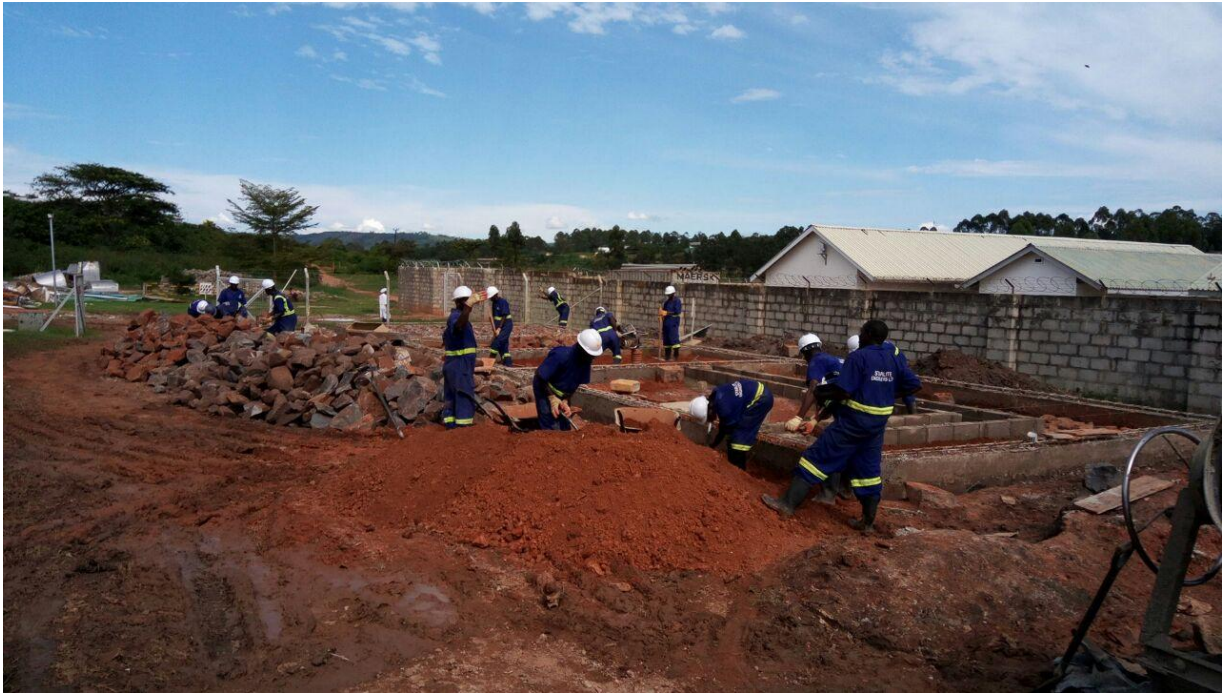
Equipment Room foundation works in progress – Coca Cola Mbarara Plant
