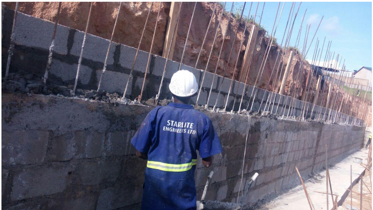
Retaining wall for equipment slab – Namanve plant
