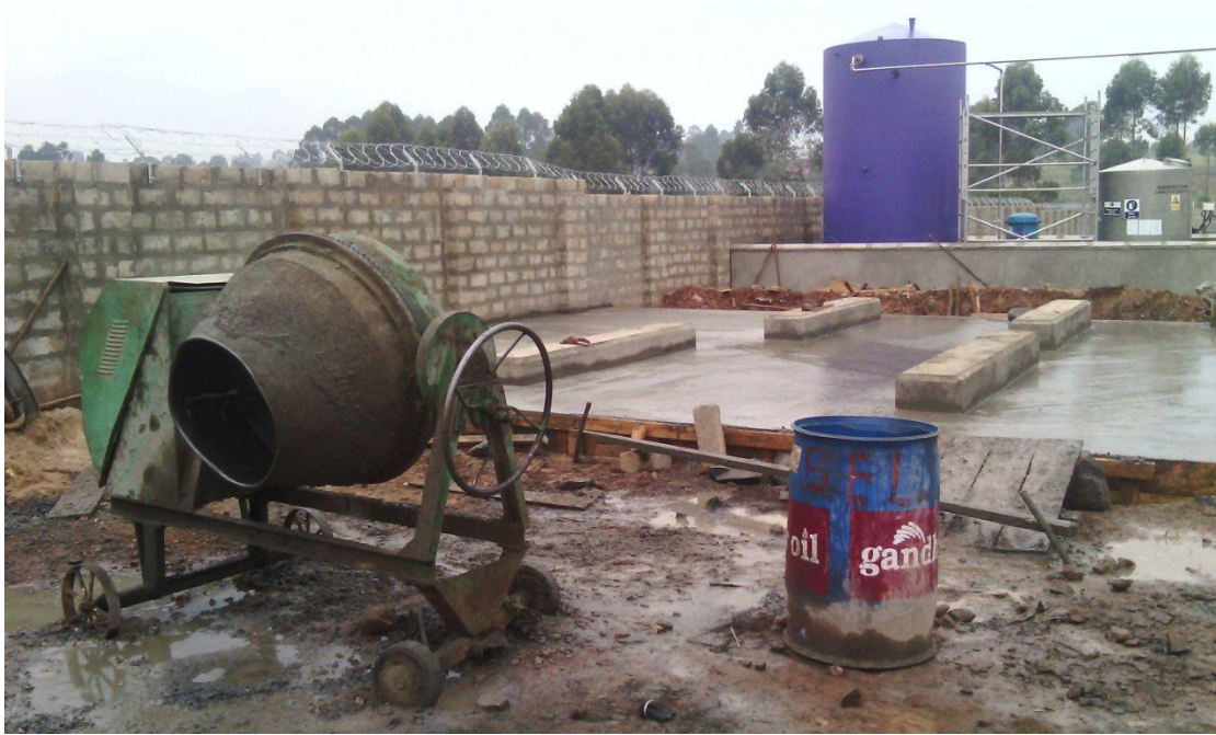
Above ground fuel tanks band wall (containment) works in progress- coca cola Mbarara plant
