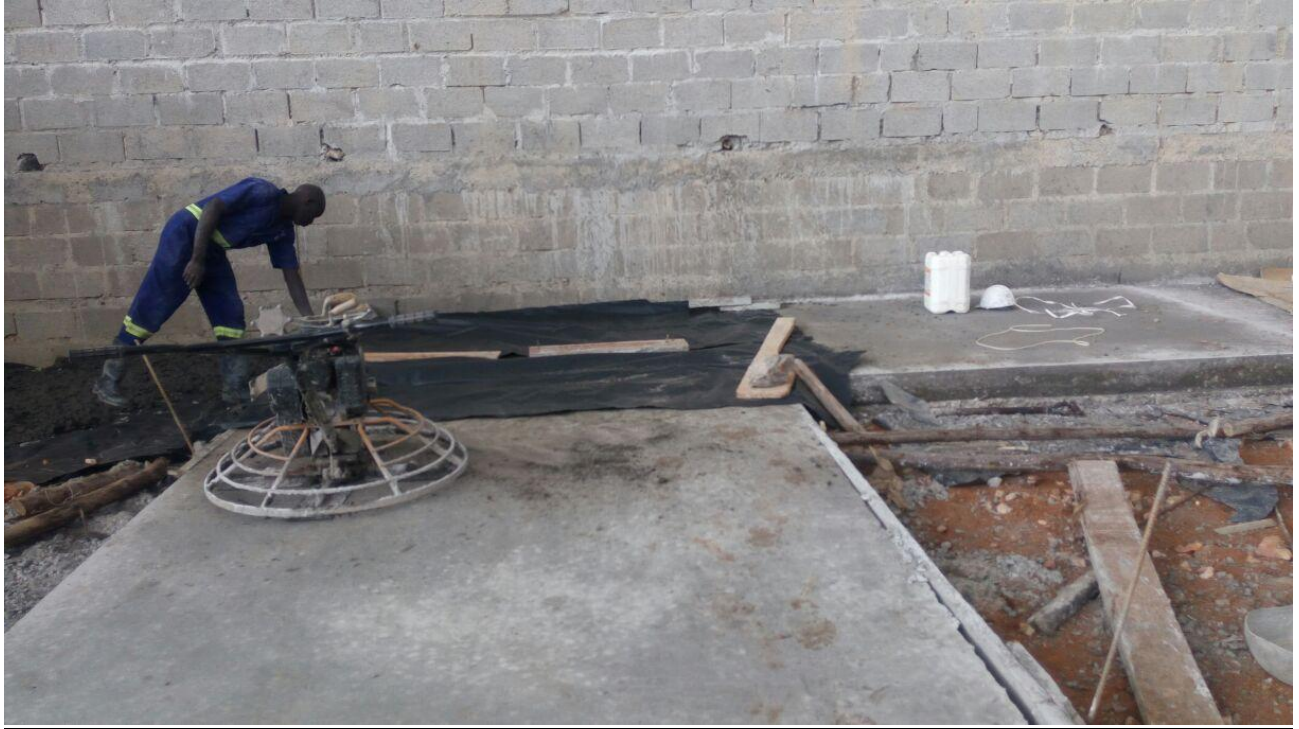
Power floating 200mm thick concrete slabs
