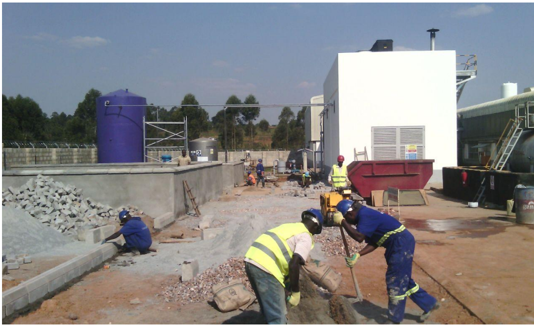
Above ground fuel tanks band wall (containment) complete- coca cola Mbarara plant
