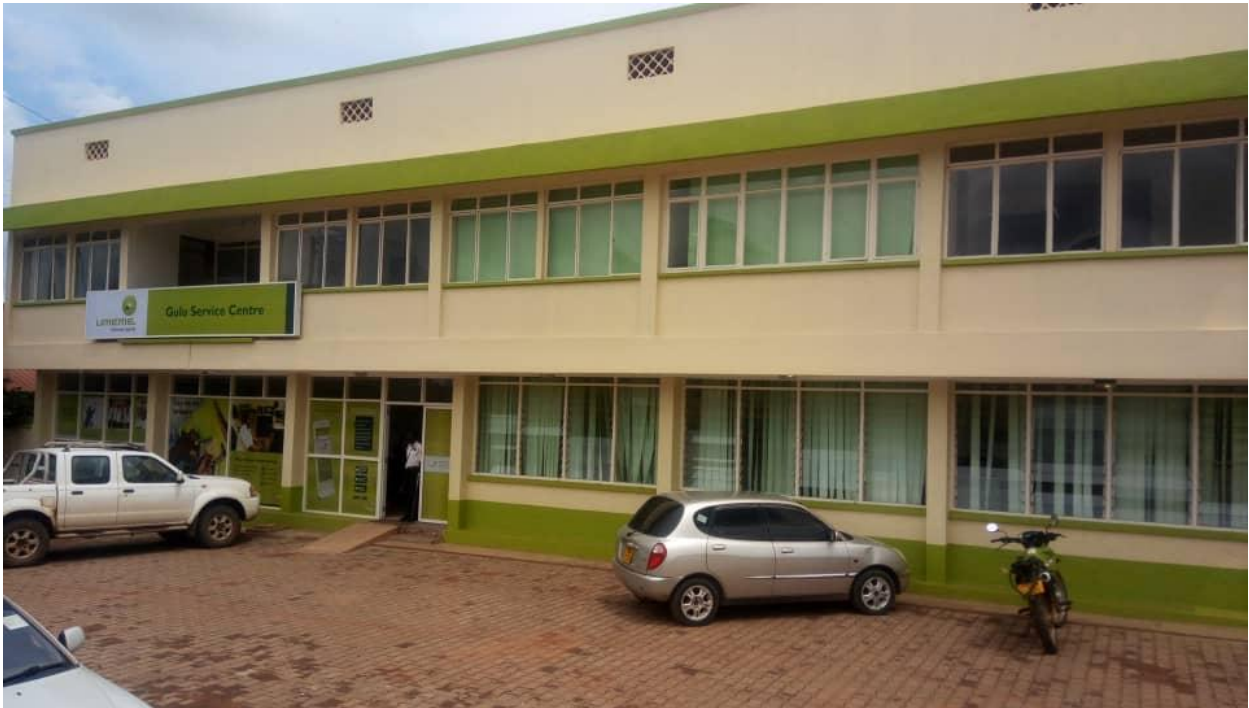
UMEME offices at Gulu after refurbishment
