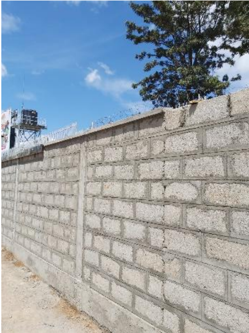
Perimeter wall block works in progress - BOU Arua Branch.
