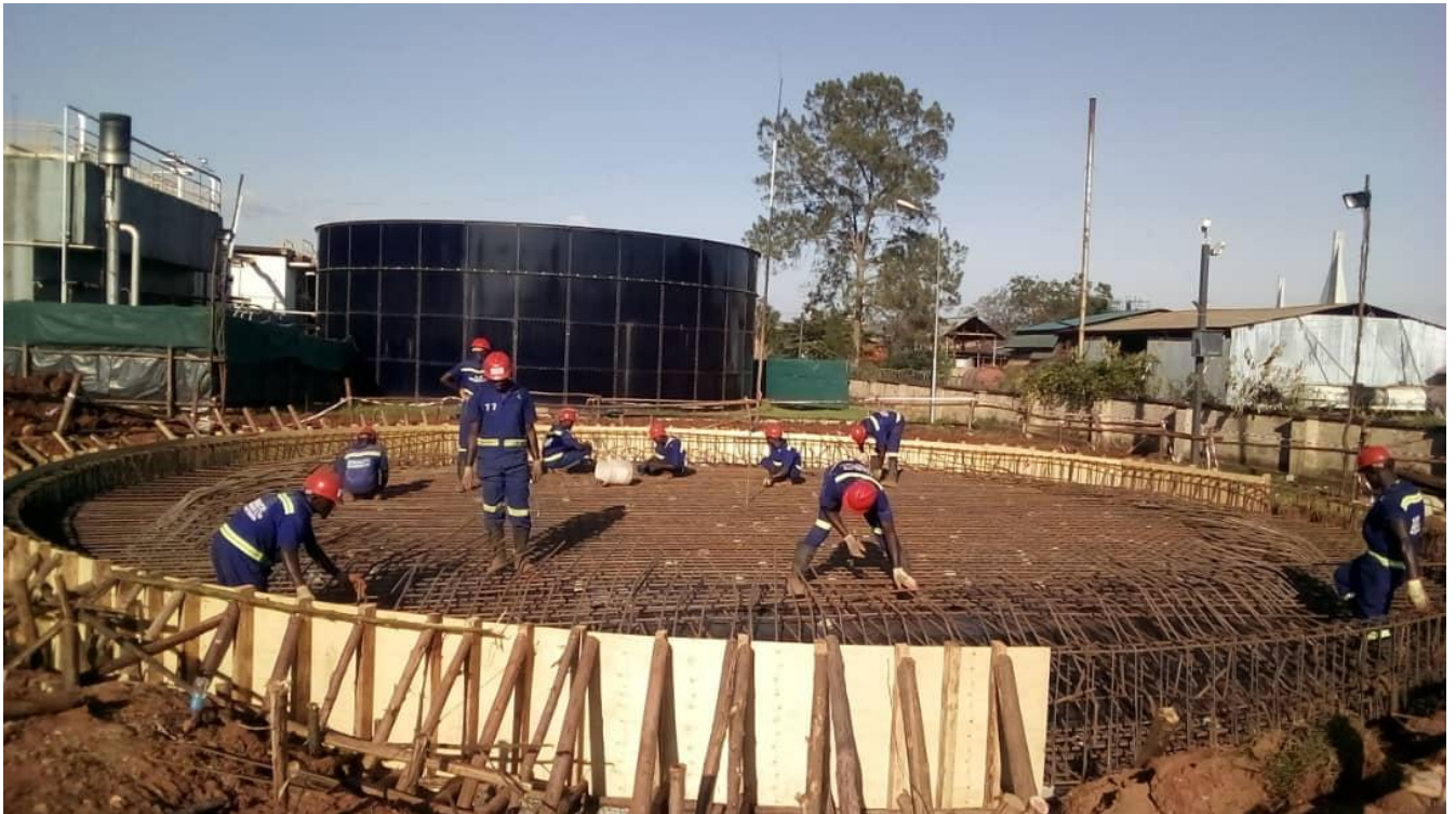
Steel work for calamity tank foundation at Nile Breweries Jinja Plant
