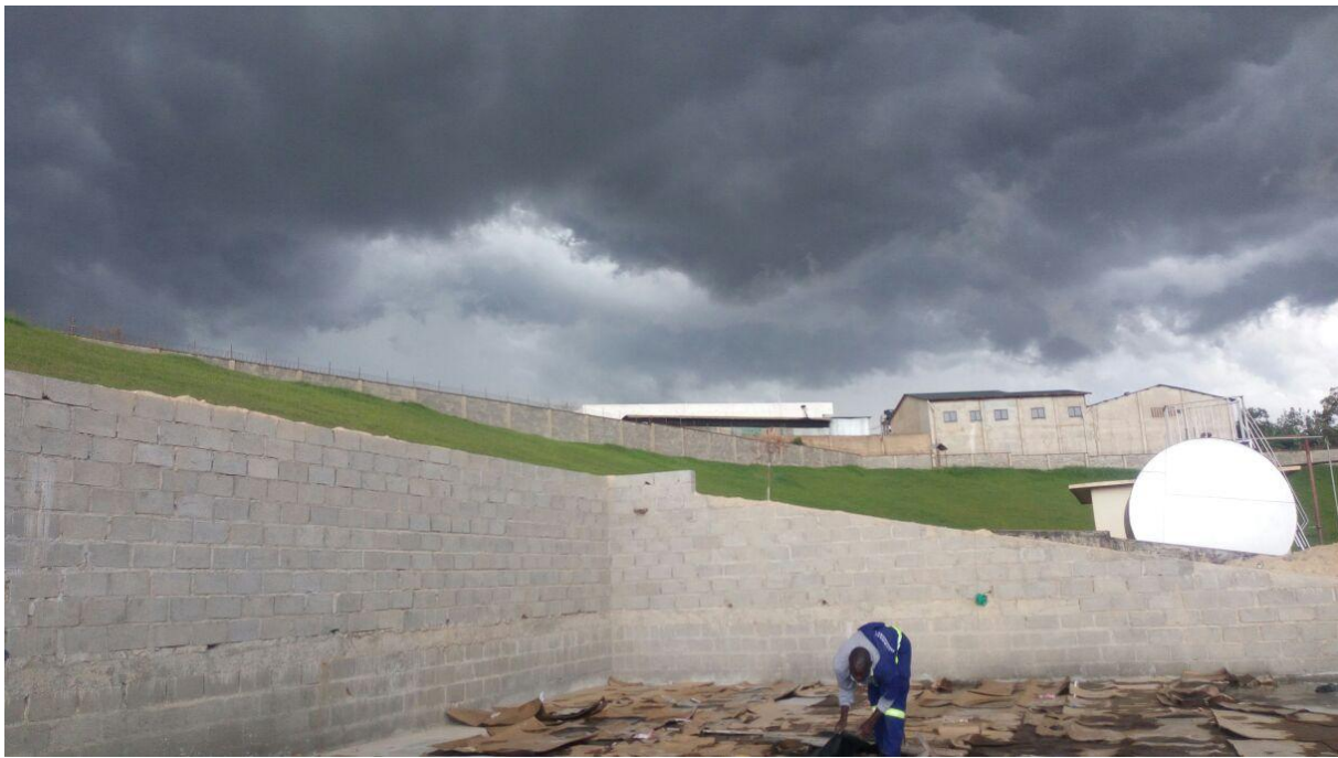
Retaining wall and slab works in progress at Coca Cola Namanve Plant
